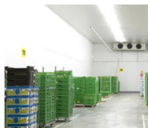
Cold Storage & Freezer Rooms
